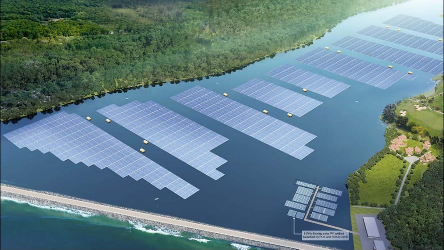
Artist impression of the upcoming 60MWp floating solar system on Tengah Reservoir. (Photo: PUB/Sembcorp)
